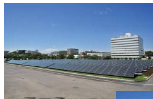
A total of 488 kW is generated from two sites: 352 kW from 1,760 PV modules (above); and another 136 kW from 680 PV modules (right).
