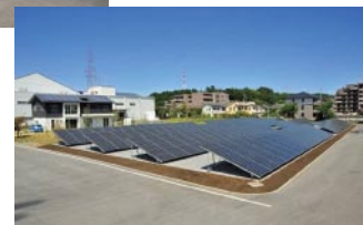
A total of 488 kW is generated from two sites: 352 kW from 1,760 PV modules (above); and another 136 kW from 680 PV modules (right).
