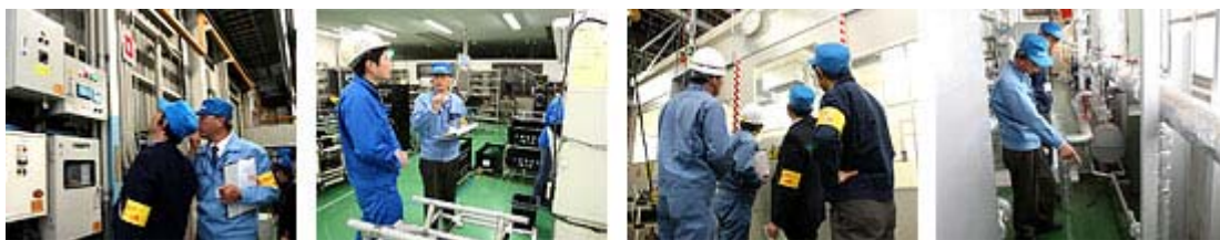
Energy conservation experts conducting inspections.
