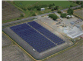
Large-scale power generation equipment
