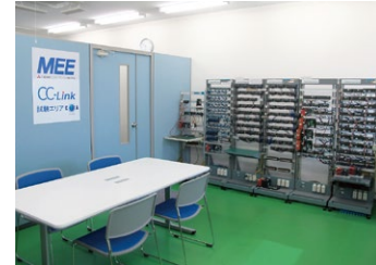
Conformance testing lab
