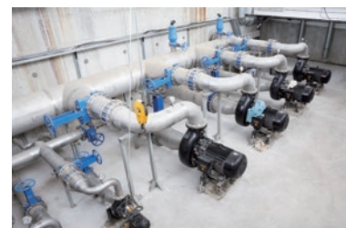
Sewage treatment plant
